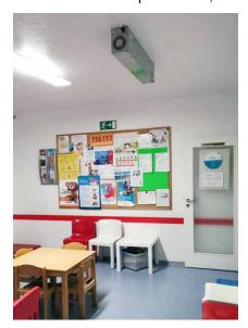
work undisturbed. In the waiting room, SteriWhite Air C was installed on the ceiling – very simply and without any problems, as Christian Baus emphasised. And that is all that is required for some time, because apart from replacing the UV lamps, no further maintenance is needed, and the lamps have a service life of up to 16,000 operating hours.
